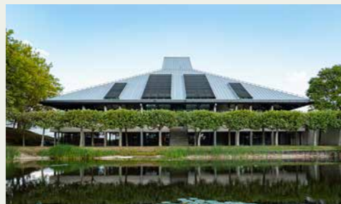
The IVC Flooring Development Centre in Waregem (Belgium) has been turned into a sustainable base. It uses heat recovery, intelligent lighting technology and is powered by solar panels on the building.
